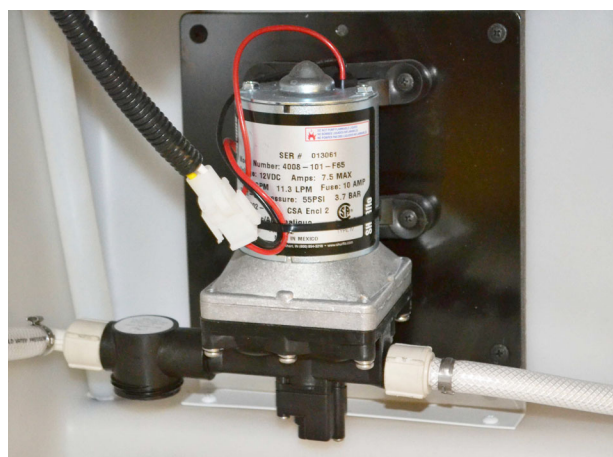
Water Pump -Typical View
