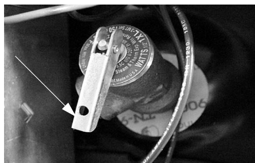
Pressure-Temperature Relief Valve (Lift handle only when water heater is cold) -Typical View
